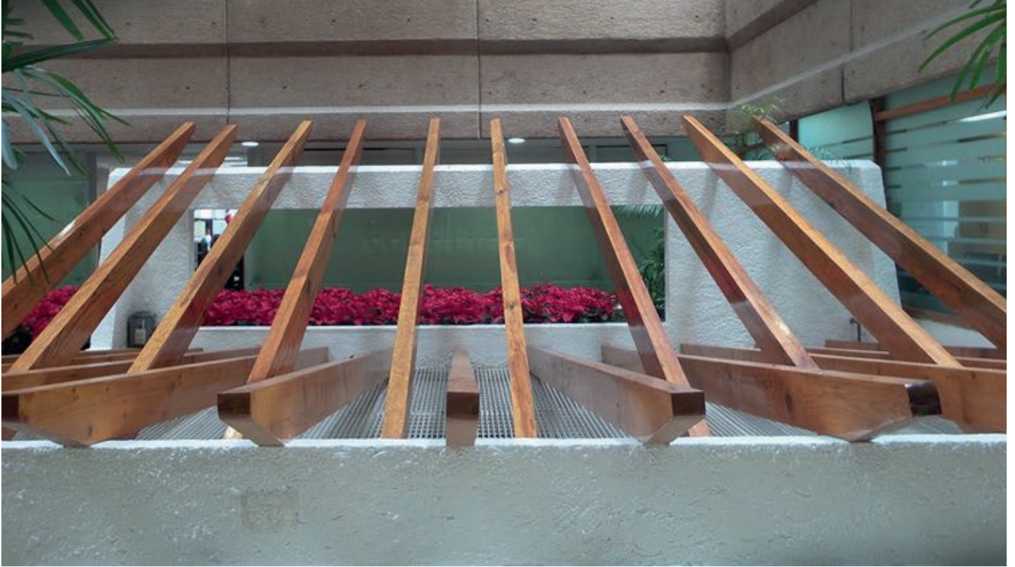
Carpentry work Ferromex Offices, Mexico City
